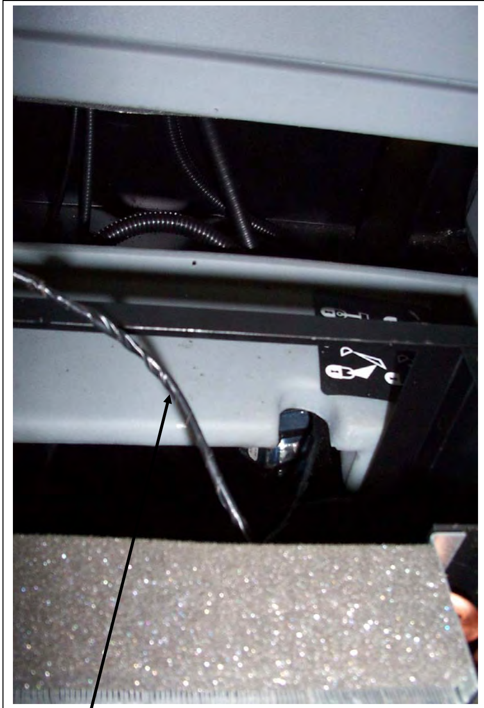
Thermostat probe run before AC coil installed
